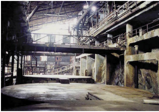
A view at the base of the Concentrator Building
