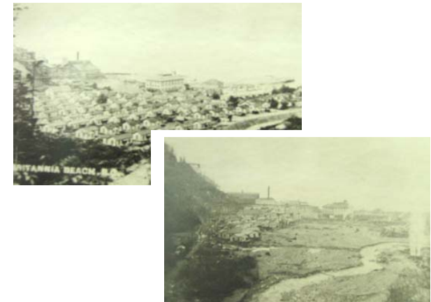
Figure 1: Before and After the 1921 Debris Flood (Source-BC Museum of Mine Mining)
