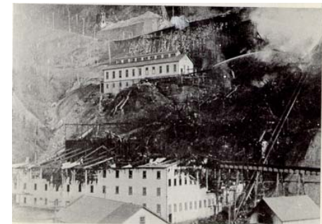
The remains of the Concentrator Building after the fire of '21. Photo from Ramsay, Bruce, Britannia: The Story of a Mine , Agency Press Ltd., Vancouver 1967
