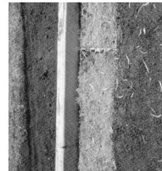
Figure 1-3 and 1-4 - Curb system captures stormwater where it falls, encouraging water retention and infiltration.
