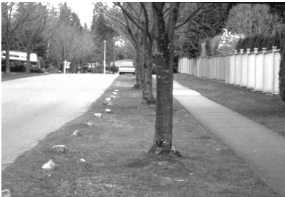
Figure 4-1 - Streets were edged with a grassy shoulder enabling infiltration capacity at the roadside, an essential aspect of the overall stormwater system.
