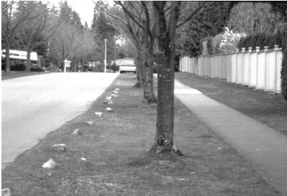
Figure 4-1 - Streets were edged with a grassy shoulder enabling infiltration capacity at the roadside, an essential aspect of the overall stormwater system.
