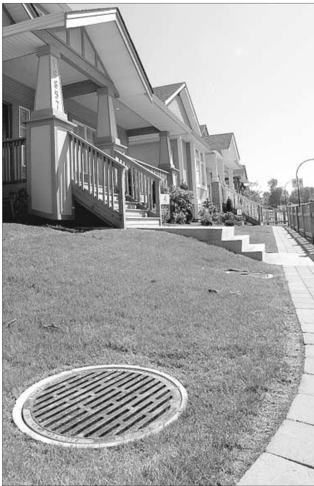
East Clayton homes are equipped with dual drainage systems: crushed rock pits under the lawns that hold and store rain water, and storm sewer connections to handle any overflow.
