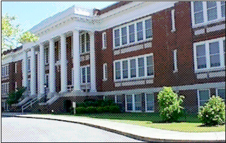
SCHOOL CONVERSION: This former school in Edenton, featuring an elegant colonnaded entrance, was preserved, but the use changed. It is now an apartment building. Maintaining historic schools as schools can promote the walkable neighborhood school concept because they typically are within walking distance of older residential areas. They also reduce the need for new schools.
